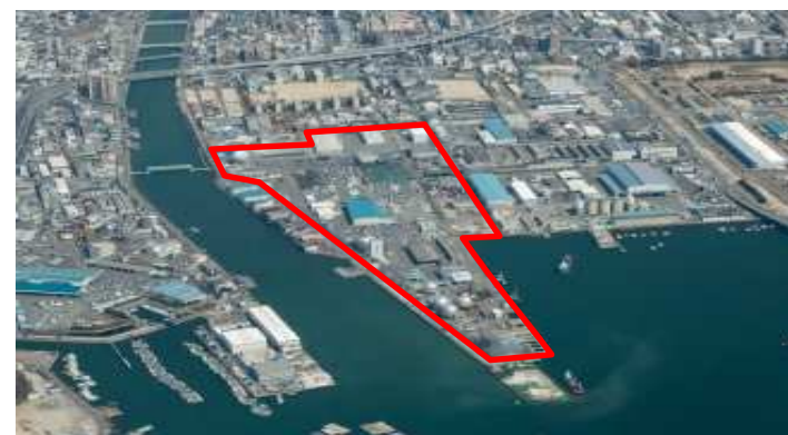
Planned site of the new power plant
