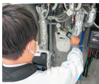
Safety inspection of gas equipment
