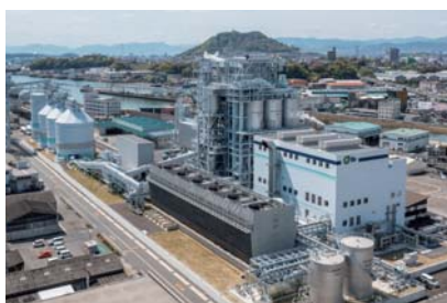
Kaita Power Station (biomass generation)
