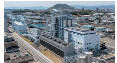
Kaita Power Station <Kaita Biomass Power> (Myojinmachi, Kaita Town)
