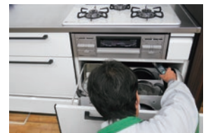
Safety inspection of gas equipment
