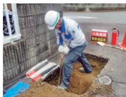
Gas piping work
