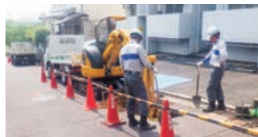
Gas piping work
