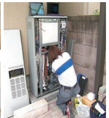
Maintenance of an "Ene-Farm" household fuel cell
