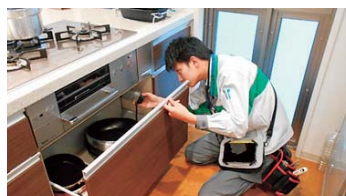
Safety inspection of gas equipment
