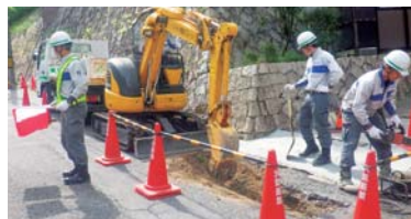
Gas piping work
