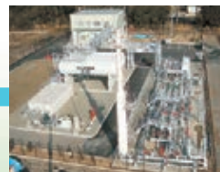
Mizushima station (Setouchi Pipeline Co., Ltd.)
