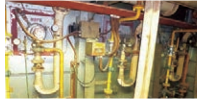
Gas industrial furnace
