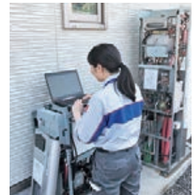
Maintenance of an "Ene-Farm" household fuel cell
