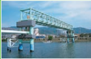
Gas pipe bridges
