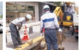
Gas piping work
