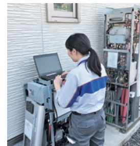
Maintenance of an "Ene-Farm" household fuel cell
