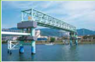
Gas pipe bridges
