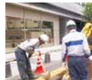
Gas piping work
