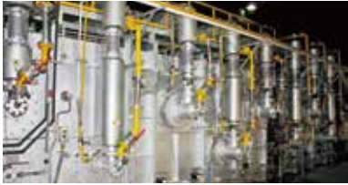
Gas industrial furnace
